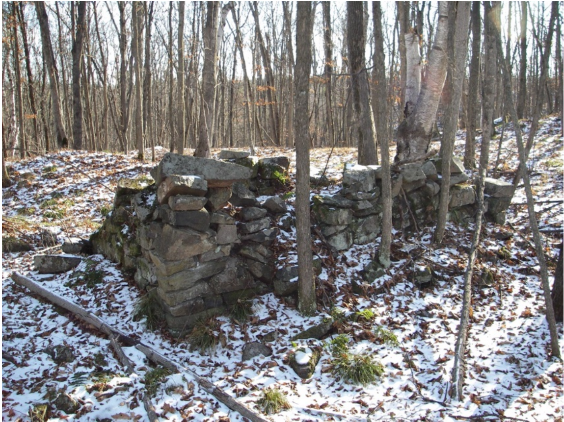
Remains of structure associated with the Bell and Claxton Mine – located to east of the opening Frank Phelan photo Nov 2008
