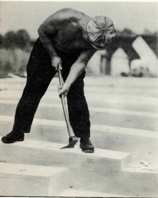
Expert workmen are employed to build the great doors of the locks.
